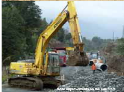
Road improvements on the Carretera
